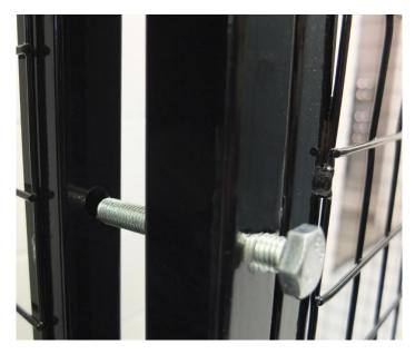
2. Place the first **side panel** against the rear panel, aligning the bolt holes. Fix with the bolts and nuts provided, ensuring nuts are fixed on the **inside**. Repeat on the opposite side.
