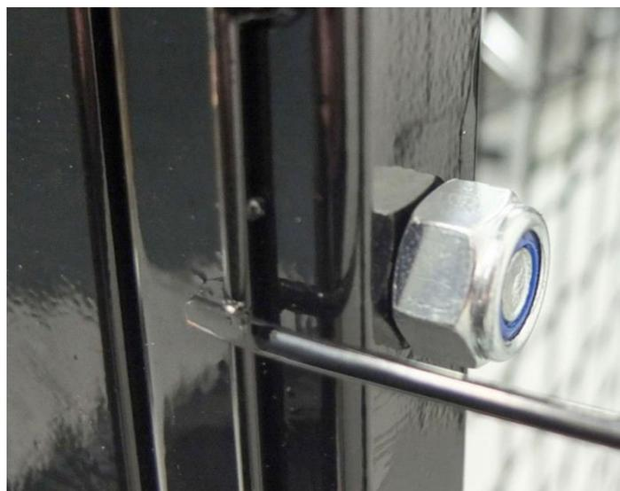
3. Offer the **door panel** to the side panels. Again, align the bolt holes and fix with the bolts and nuts provided. Ensure that the bolts are tight!
